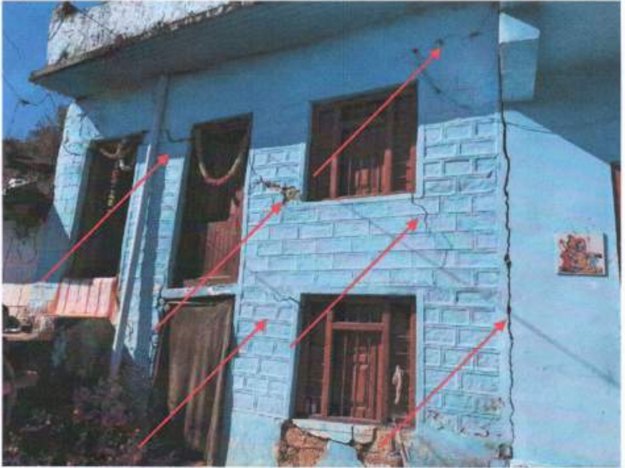
Lateral Cracks appearing in a House in Village Kande Kanyal These Houses are tilting towards front due to land subsidence due to the mining activities carried out on the downward slope of the hill.
