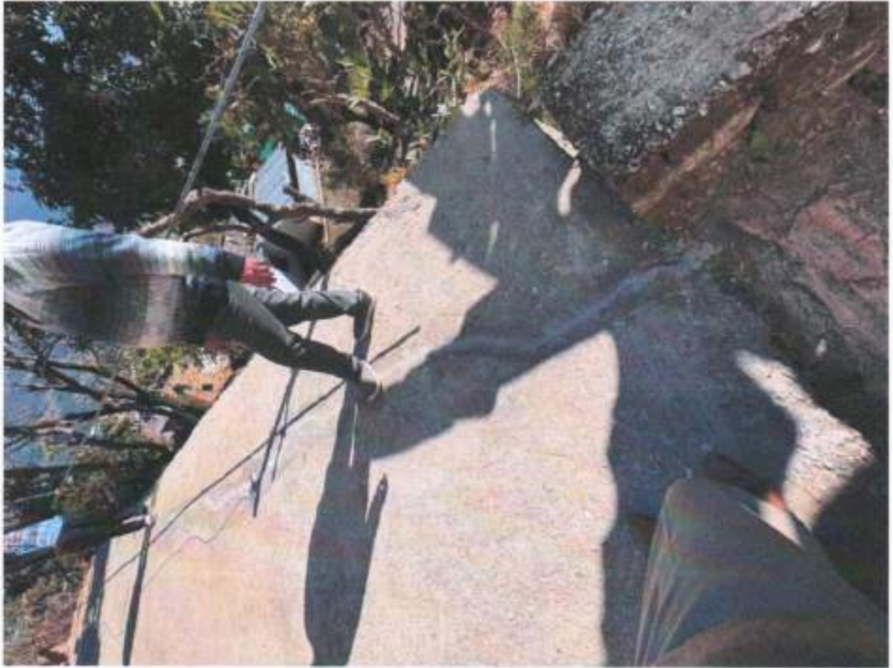
Cracked Floor in front of House in Village Kande Kanyal (UP) Cracked Staircase from Lintel Slab of House in Village Kande Kanyal (DOWN)
