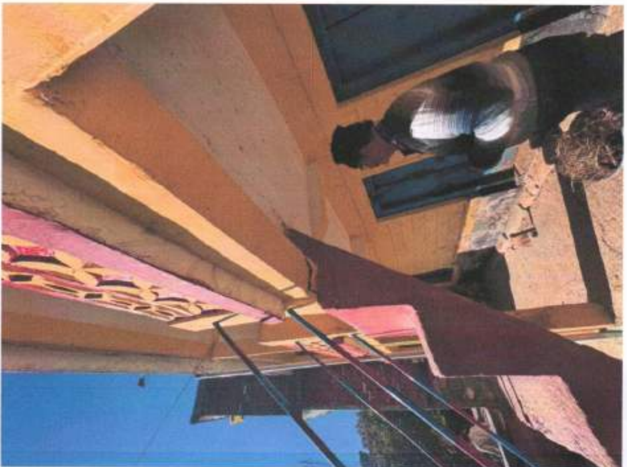
Cracked Floor in front of House in Village Kande Kanyal (UP) Cracked Staircase from Lintel Slab of House in Village Kande Kanyal (DOWN)
