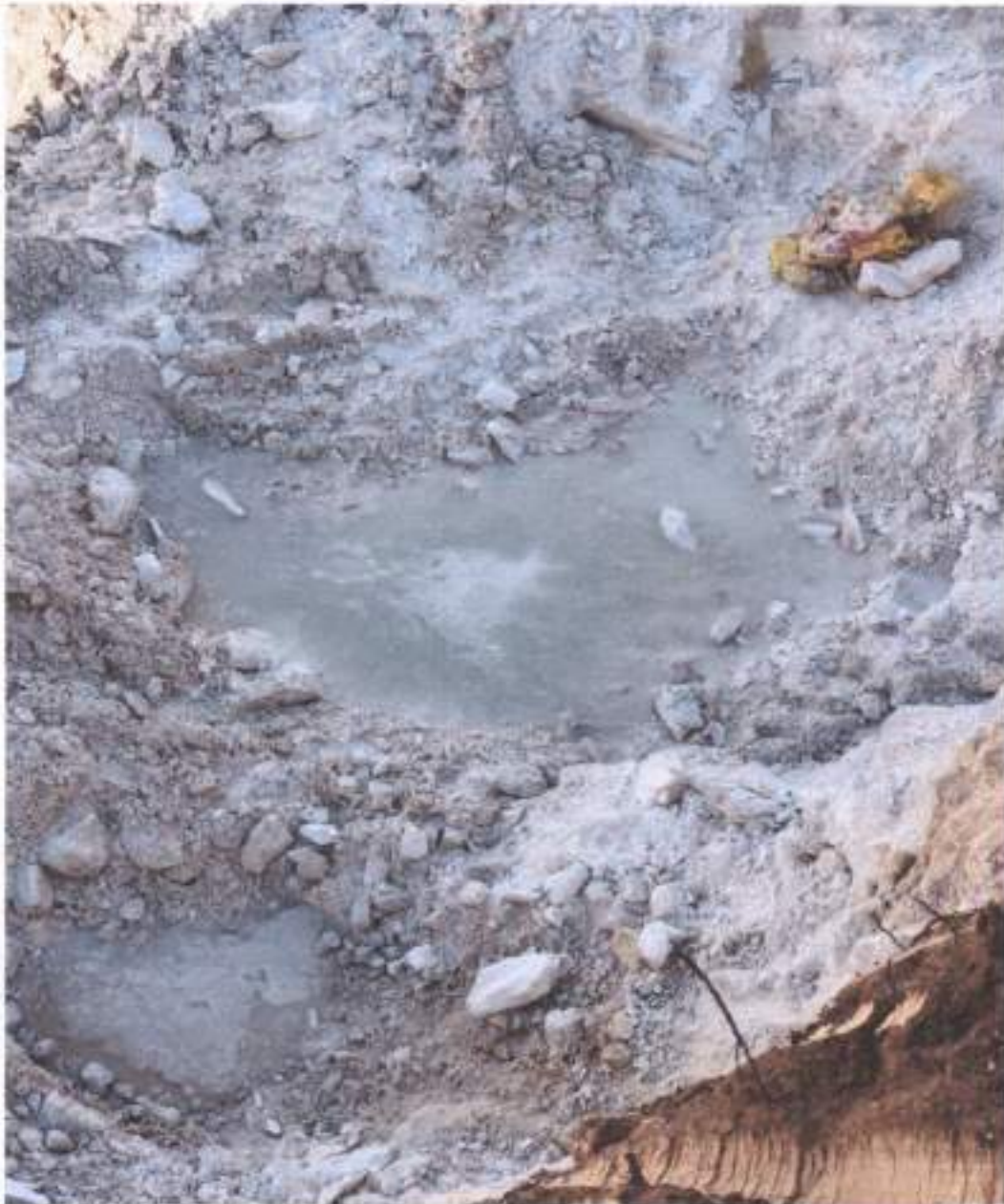
Large Water Holes with no drainage In the Mine at Village Surkali Owned by Thakur Singh Gariya Clicked from 29° 54' 45.672" N 79° 57' 14.898" E
