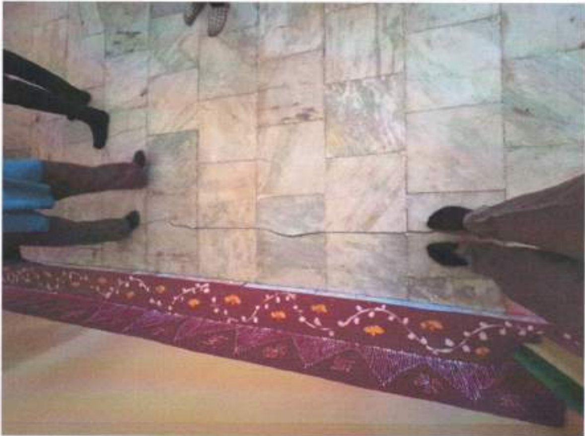
Sanctum of the temple is tilting towards left (UP) Lateral Cracks on the Floor around Temple (DOWN)
