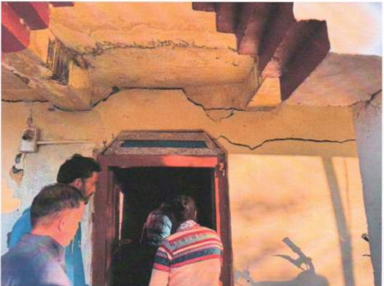
Settling of Front Porch of the Bakhli of Sri. Kandpal Failure of Beam/Lintel
