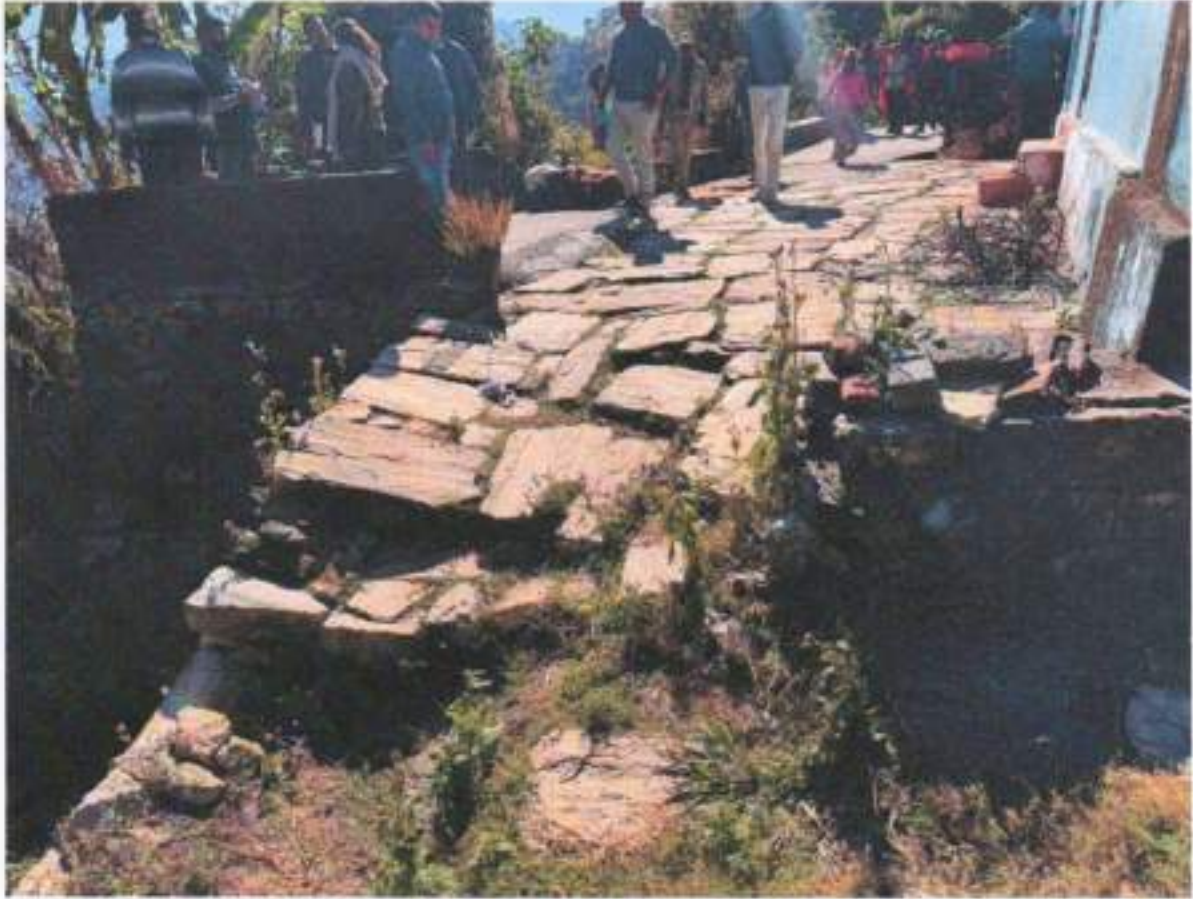
Settling of Front Porch of the Bakhli of Sri. Kandpal Failure of Beam/Lintel
