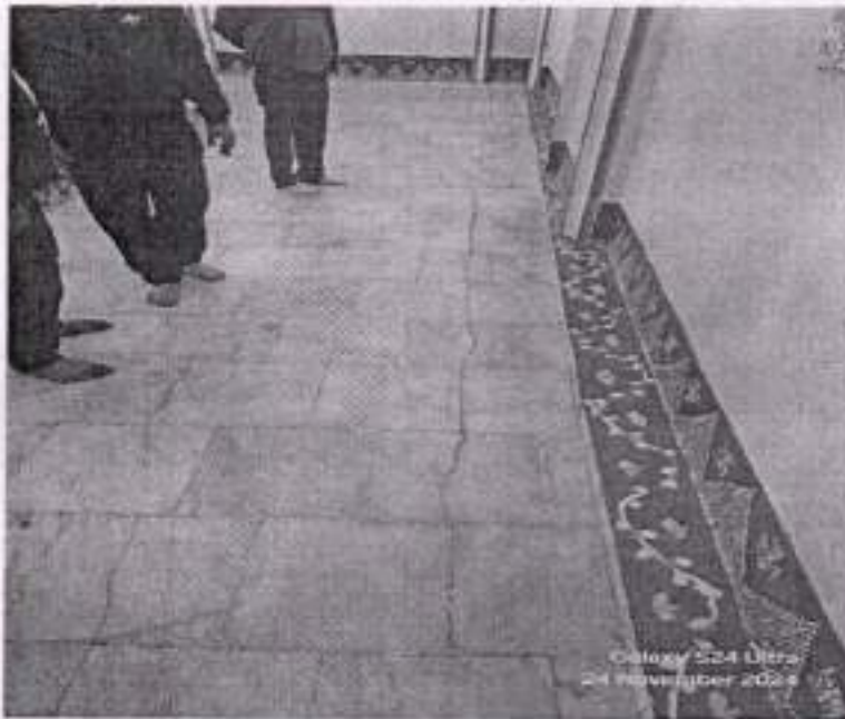
Photo 3- Cracks in flooring of Kalika Temple
